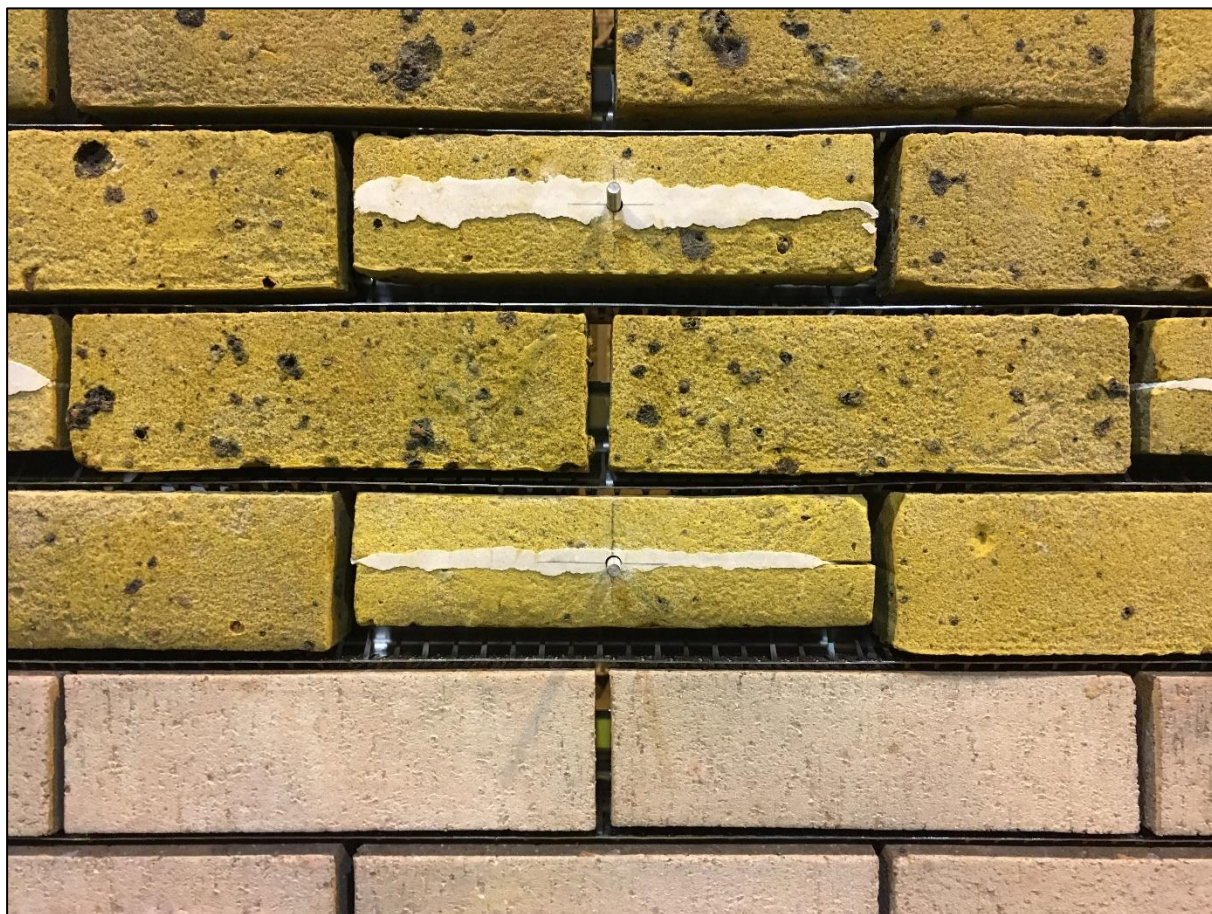
CLOST UP OF STUDS USED TO APPLY LOAD TO BRICK SLIP
