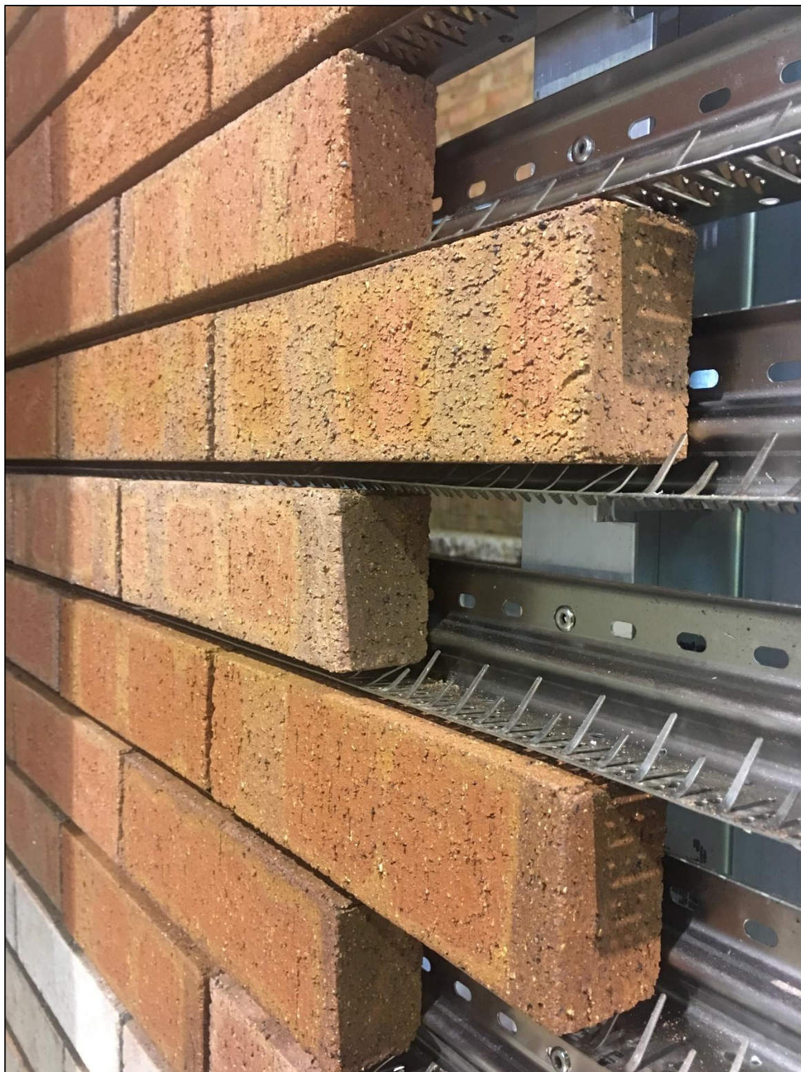
CLOSE UP OF BRICK SLIPS
